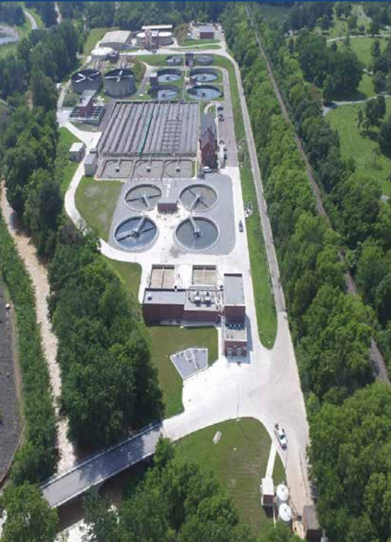
PHOTO 1: Aerial View of Lima WWTP
