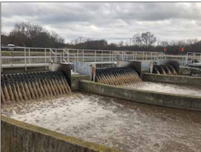
Oxidation Ditch with Disc Aerators
