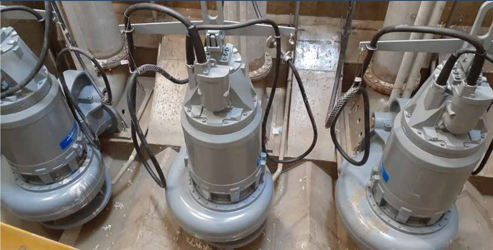
Photo 2: The three installed 15 MGD Flygt pumps (Peterson Construction)
