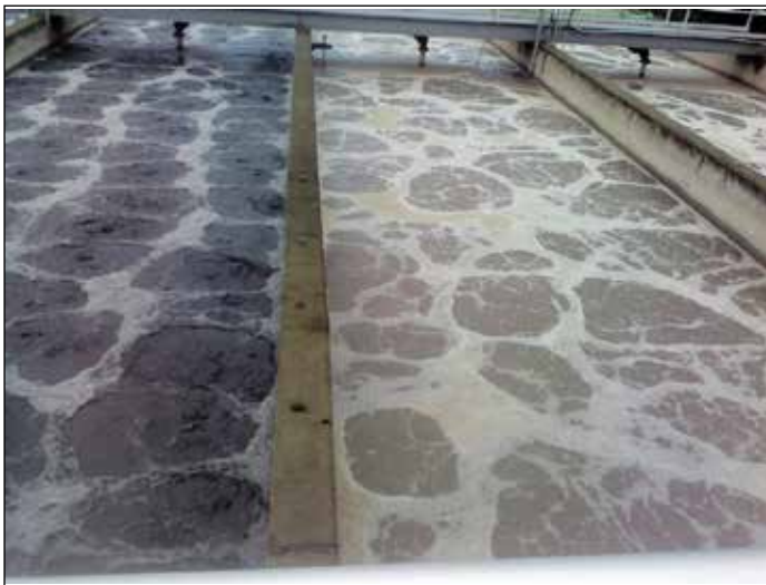
Figure 1: Isolated tank with low DO wastewater on the left and a partially recovered tank on the right
