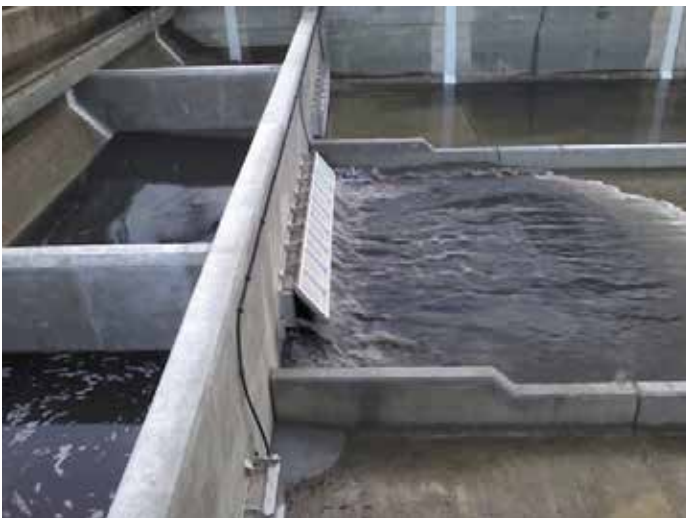
Photo 1: Flushing Gates (Stantec)
