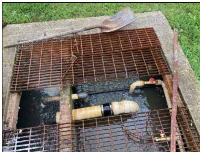
Figure 5: Portion of the package plant that served a restaurant
