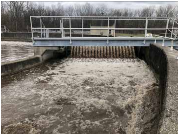
Oxidation Ditch Exterior Channel
