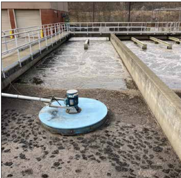
Figure 6: View of one of the anoxic zones with denitrified sludge floating on the surface
