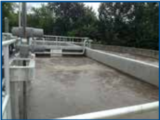
Indian Creek Wastewater Treatment Plant
