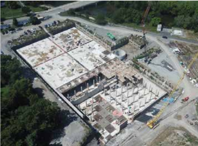
Photo 2: Aerial View of CSO Basin being built (Peterson Construction)
