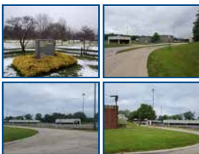
Lake County Department of Utilities - Wastewater Division
