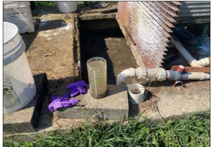
Figure 5: Note the turbid settleometer, indicating incomplete conversion
