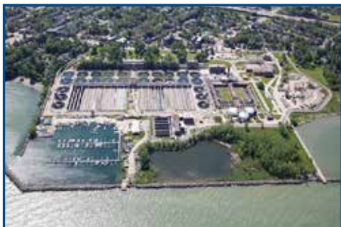
Easterly Wastewater Treatment Plant
