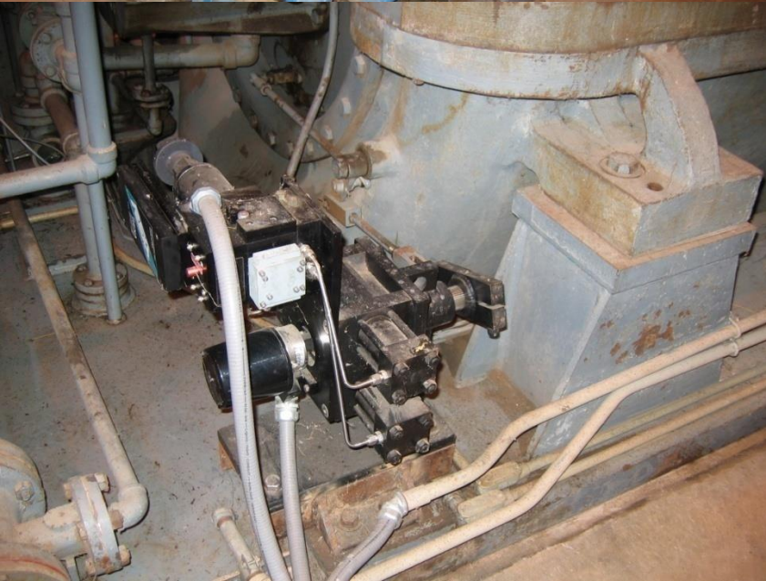
Texas WWTP Dresser Compressor Guide Vanes
