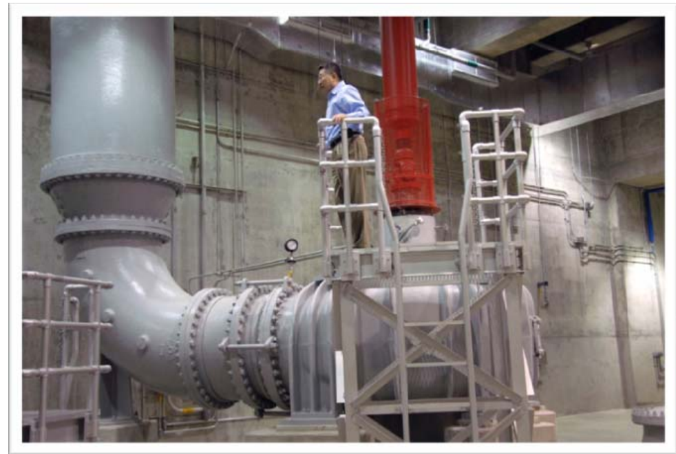
Raw Sewage Pump
