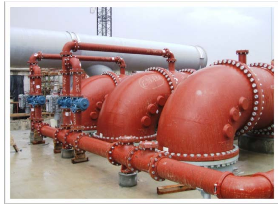
Pump Discharge Piping
