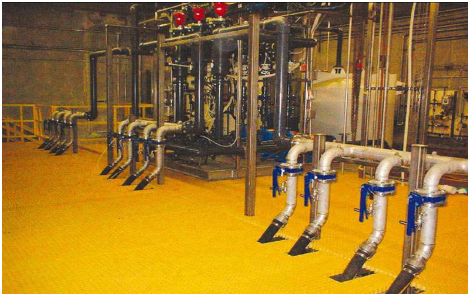
Concrete (In Ground) Membrane Tanks
