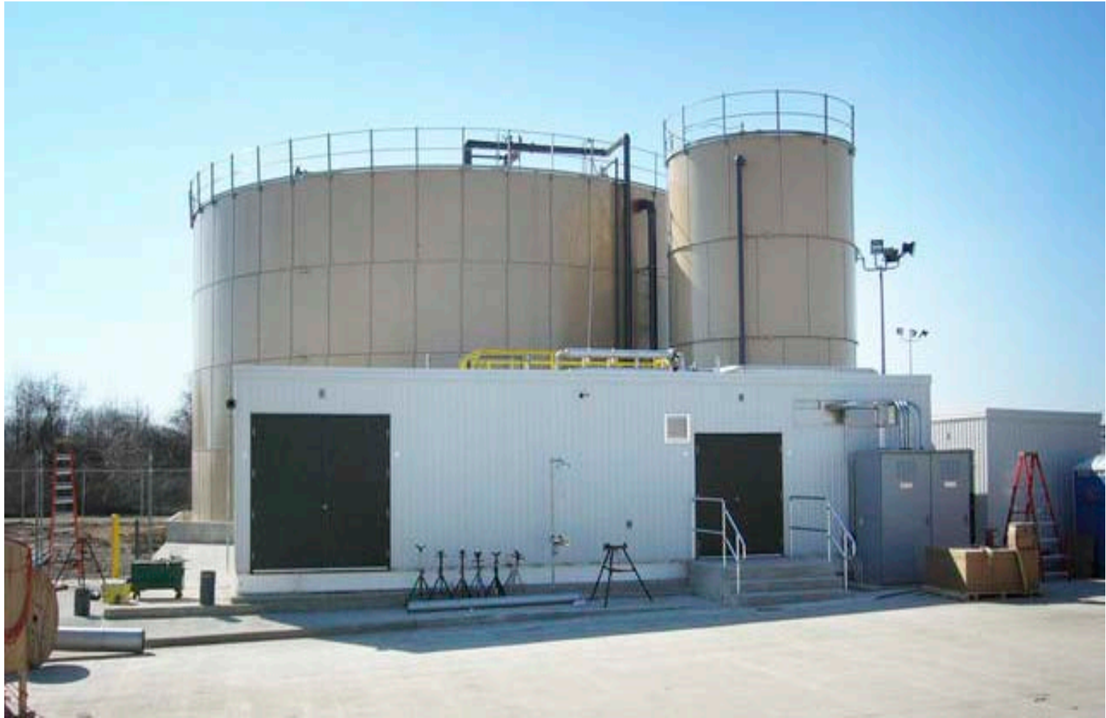
Membrane Bioreactor System
