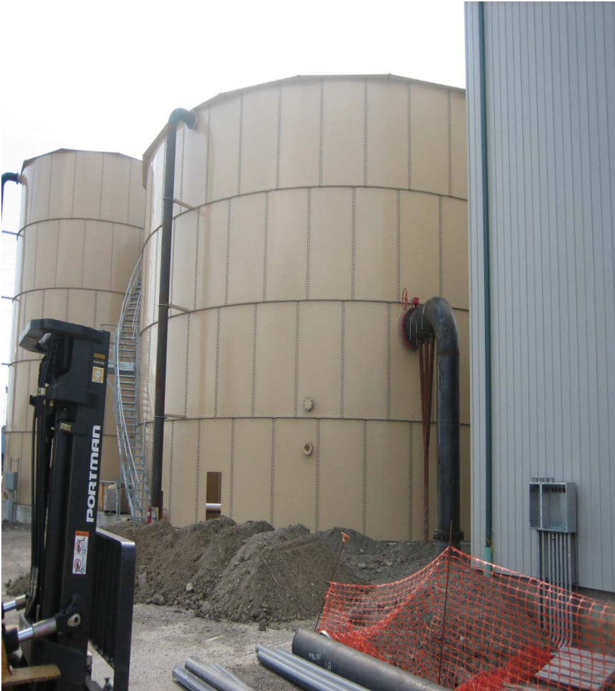
Anaerobic and Aerobic Bioreactor Tanks
