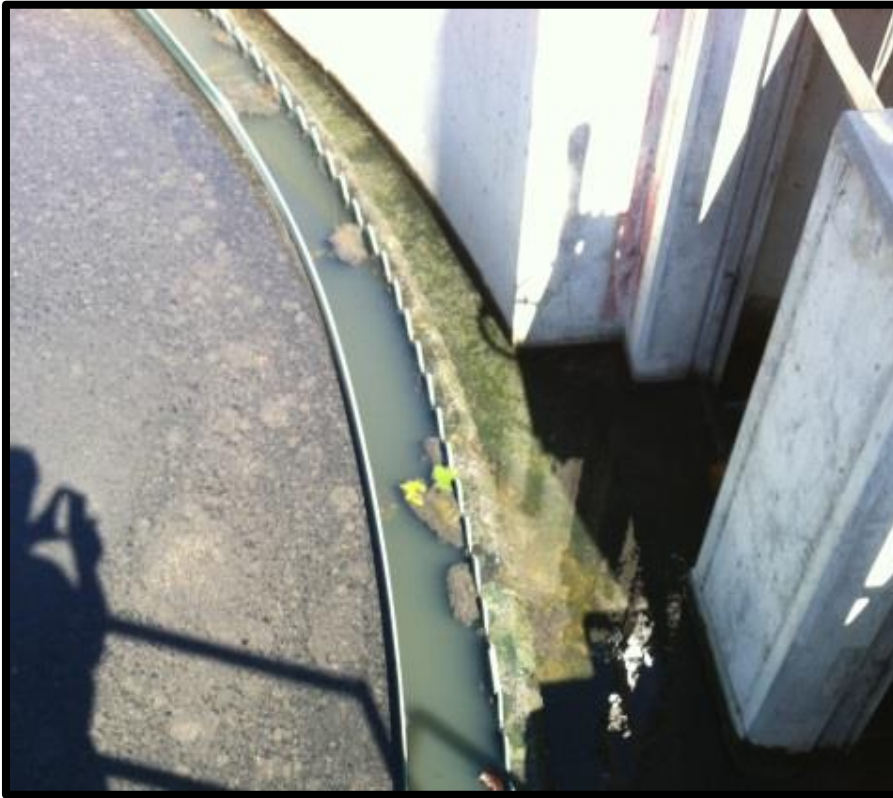
Before RE100 addition
