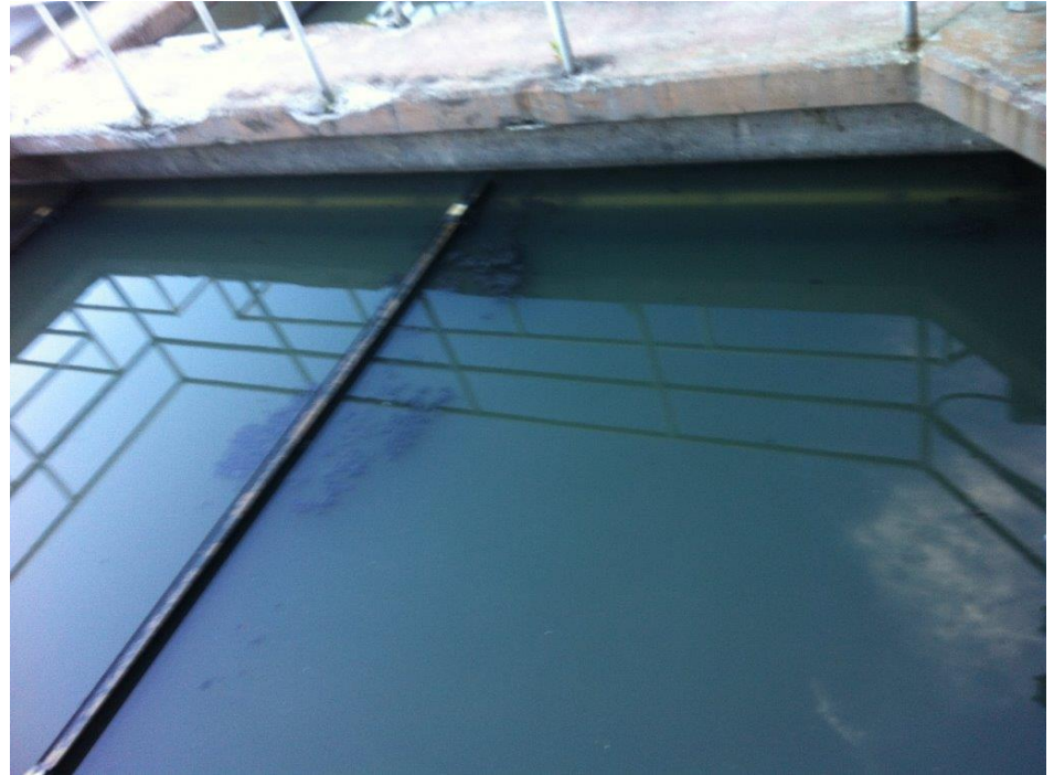
After RE 100 addition
