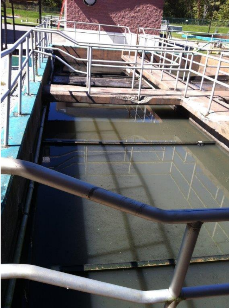
Before RE 100 addition
