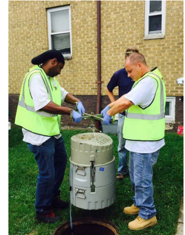
Autosampler deployed at CSO-507 sampling manhole
