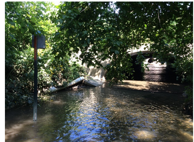
Pressure transducer installation at TR-001
