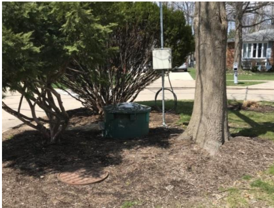
Adams Court Pump Station
