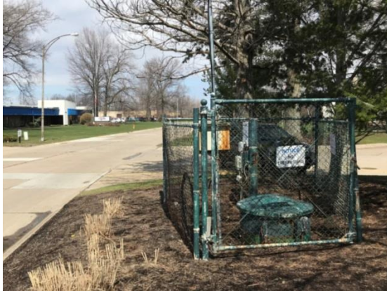
Industrial Park Pump Station
