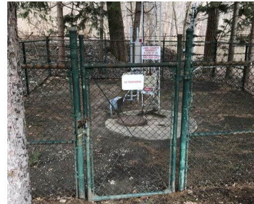
Melridge Pump Station
