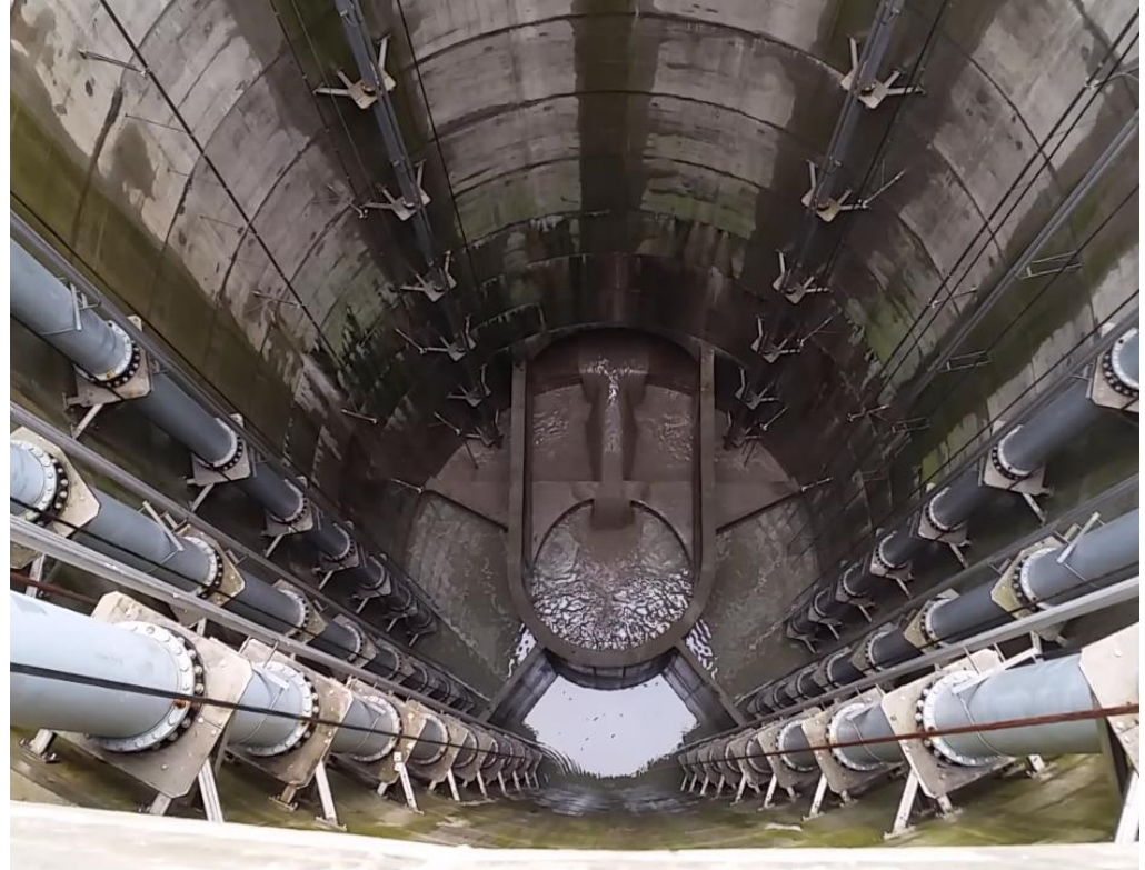
First tunnel filling test Flow enters the dewatering pumps station
