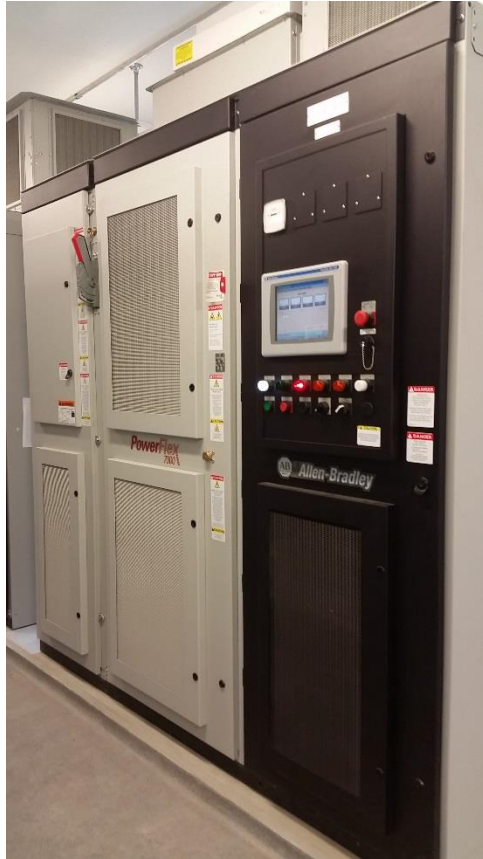
Medium Voltage Adjustable Frequency Drive
