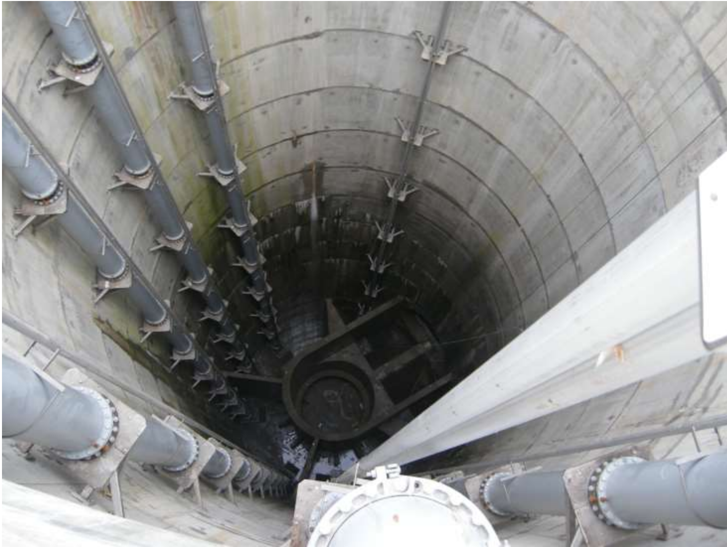
OARS Dewatering Pump Station Under Construction
