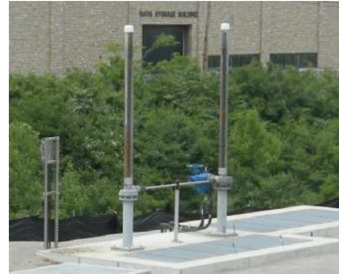
New Scioto Main Relief Weir Gate for flow balancing between plants and Southerly influent sewers storage utilization.
