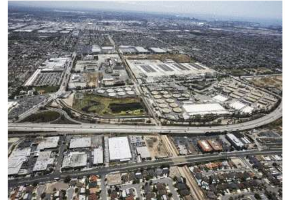
Municipal Separate Storm Sewer Systems (MS4)
