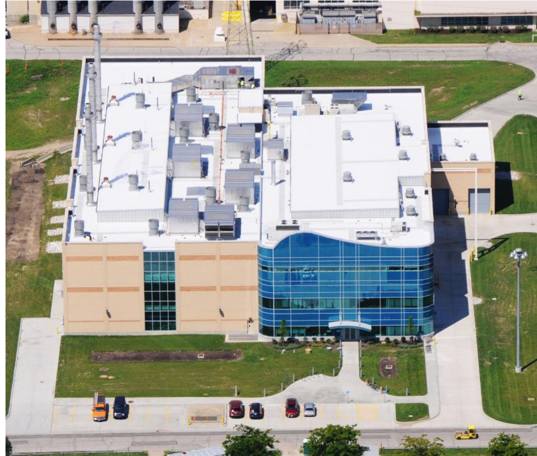
Southerly WWTC Renewable Energy Facility
