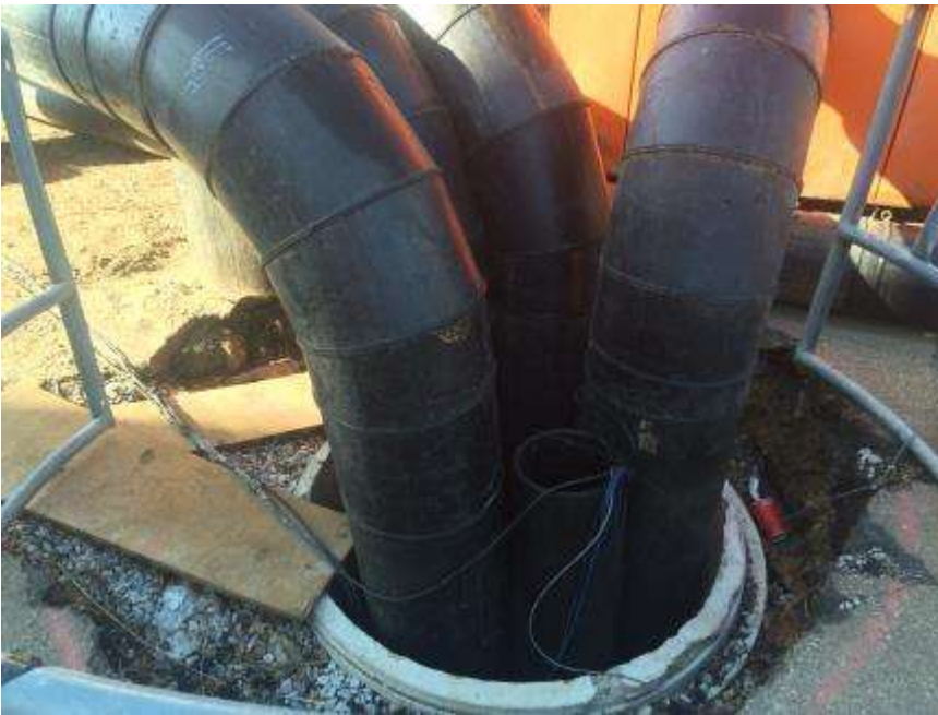
Bypass pumping suction lines
