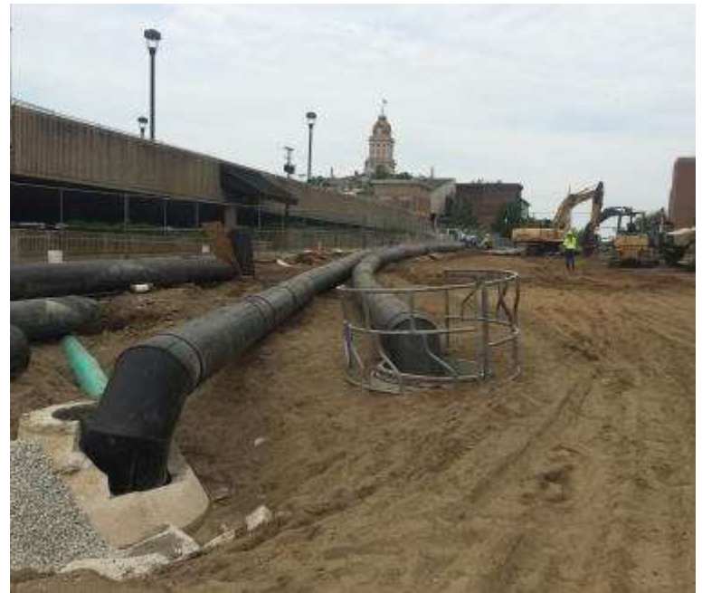
Bypass pumping discharge lines
