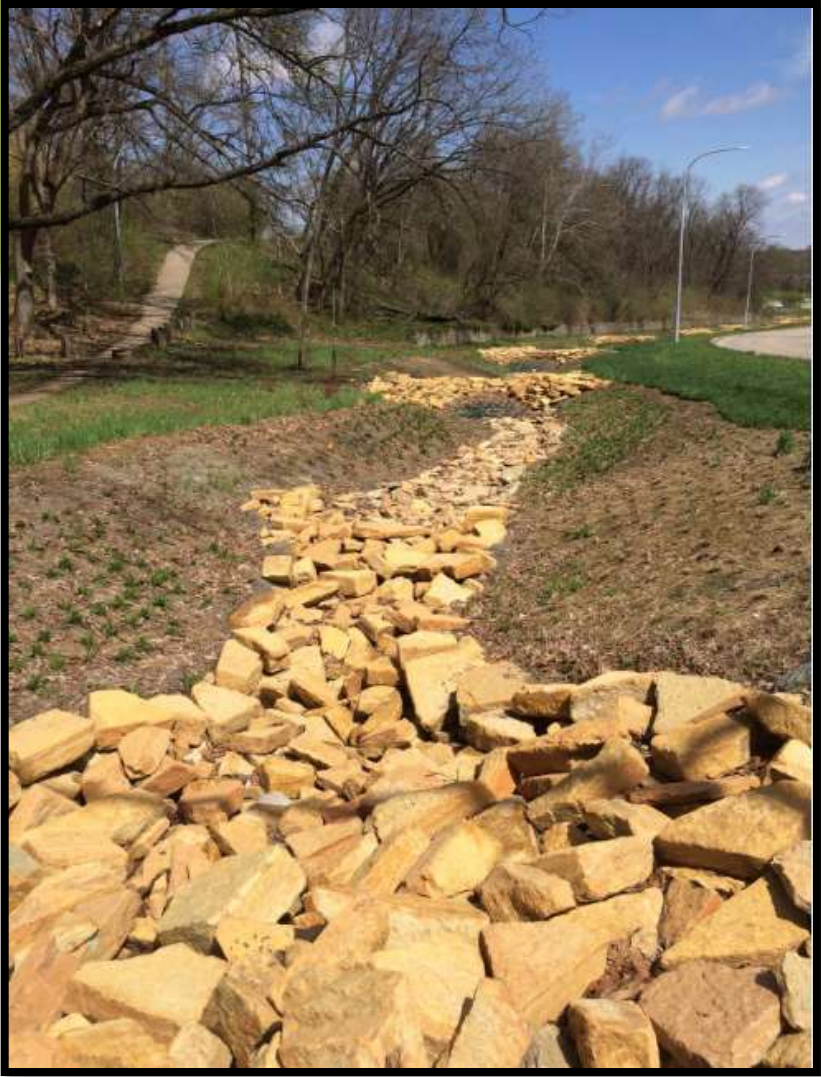
Rapid Run Bioswale
