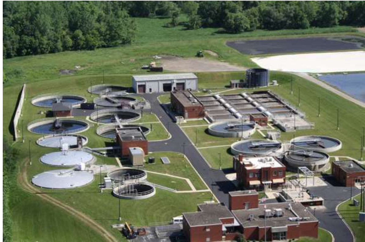
Water Pollution Control Plant Prior to quasar Project
