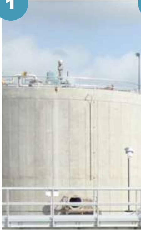
Acid Phase Digester
