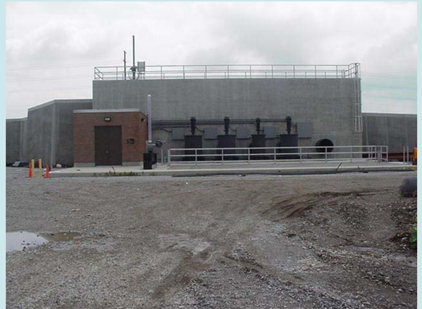
New Pump Station
