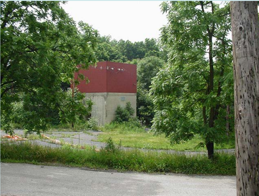
Old Pump Station
