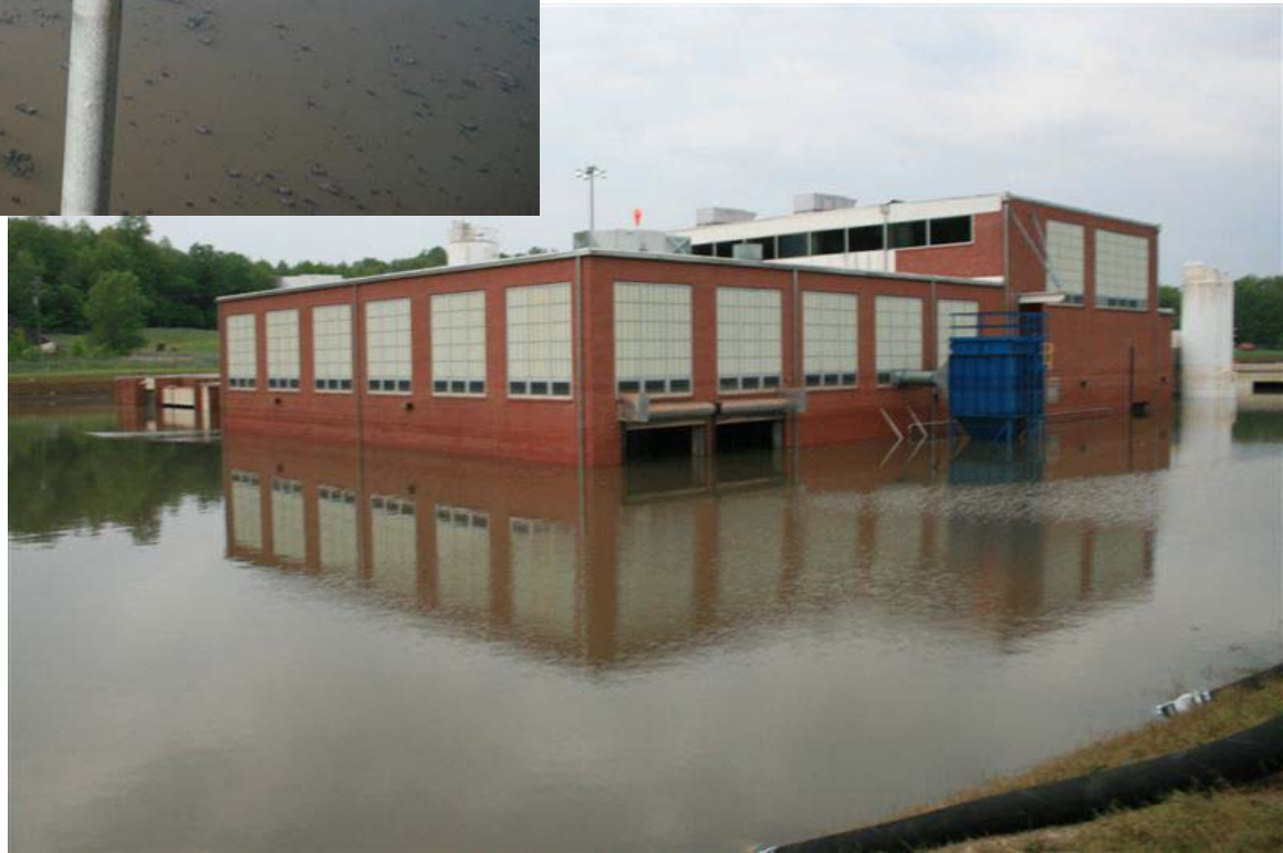
Clarksville WWTP: Solids Handling Facility May 7, 2010
