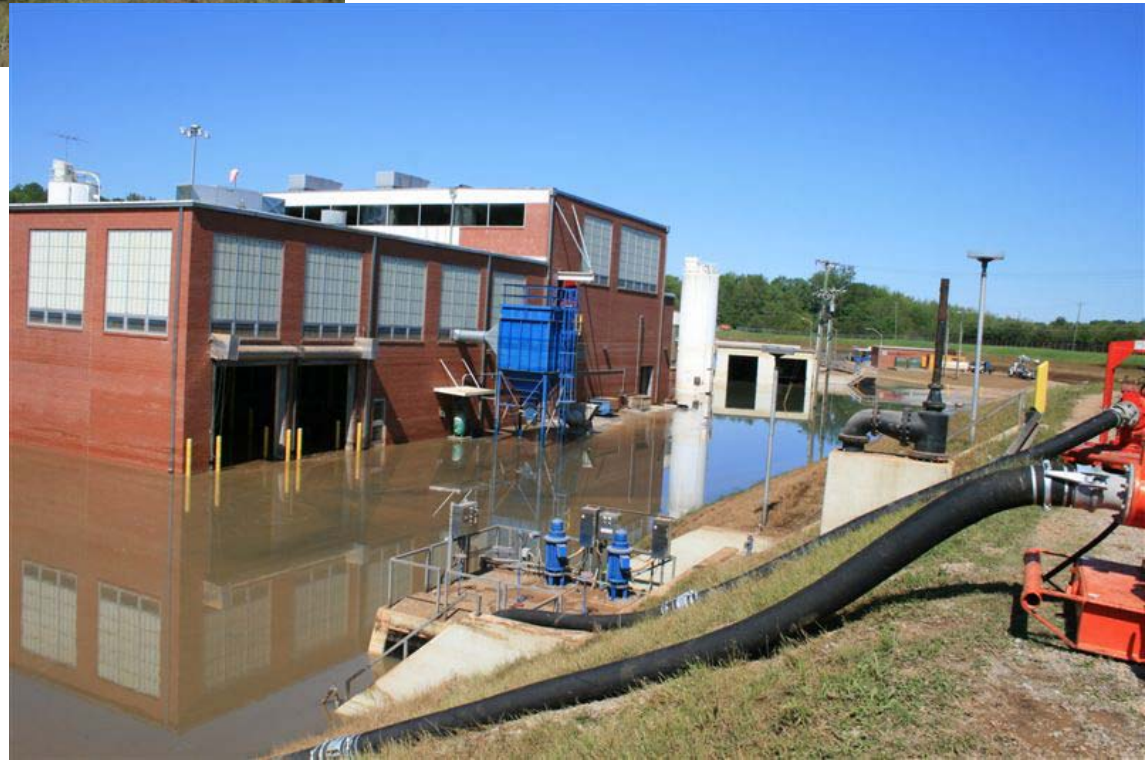
Clarksville WWTP: Solids Handling Facility May 9, 2010
